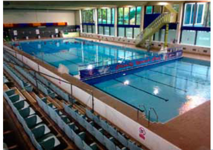
ABOVE: THE BRAMCOTE LEISURE CENTRE IS ALREADY REAPING THE REWARDS OF SWITCHING TO A HEATSAVR LIQUID COVER FOR ITS POOLS.
